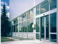
The ingenious design prevents pinching and shearing positions; emergency-OFF switches complement the safety measures. Reversing system, power limitation, speed and sensitivity of the door are immediately adjusted to the requirements at the place of implementation.
