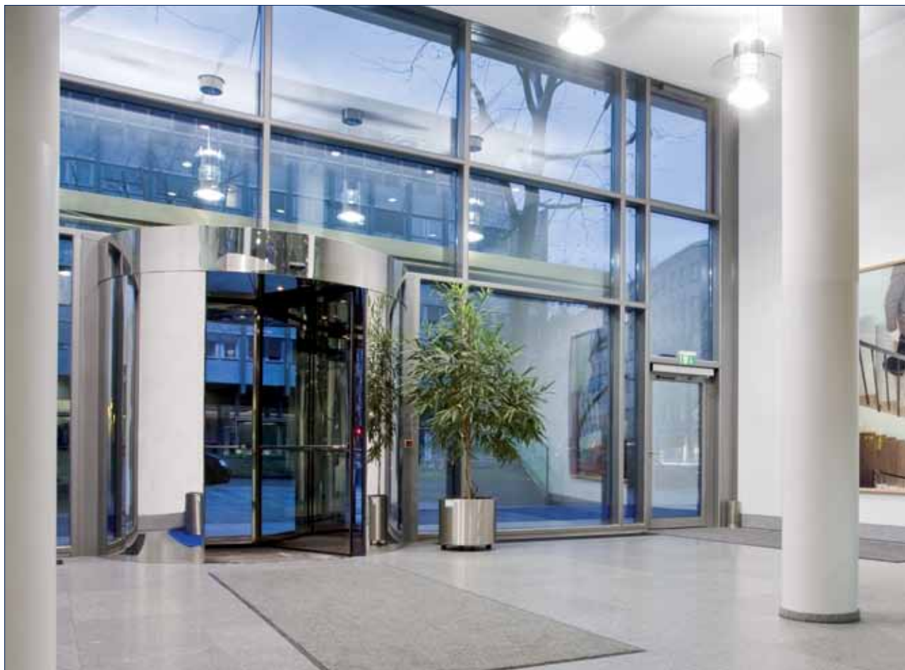
Deutsche Bank, Stuttgart · Fully-automatic GEZE revolving doors with 3 leaves and drum walls of sheet metal panels (Photo: Nikolas Grünwald)
