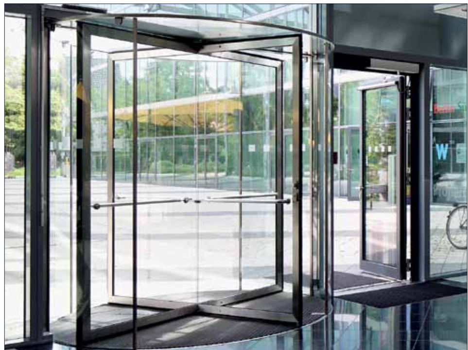
FU Campus Dahlem, Berlin Fully-automatic GEZE revolving door with 4 leaves (Photo: Stefan Dauth)
