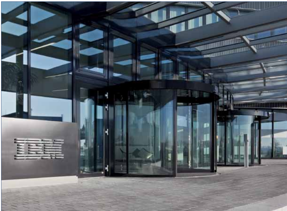
IBM Ehningen - Fully-automatic GEZE revolving doors with 4 leaves, BO function and automatic night time locking mechanism (Photo: Nikolas Grünwald)
