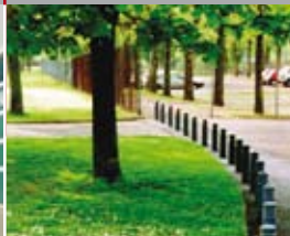
Fixed posts and bollards
