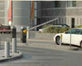
Road barriers and paying parking systems
